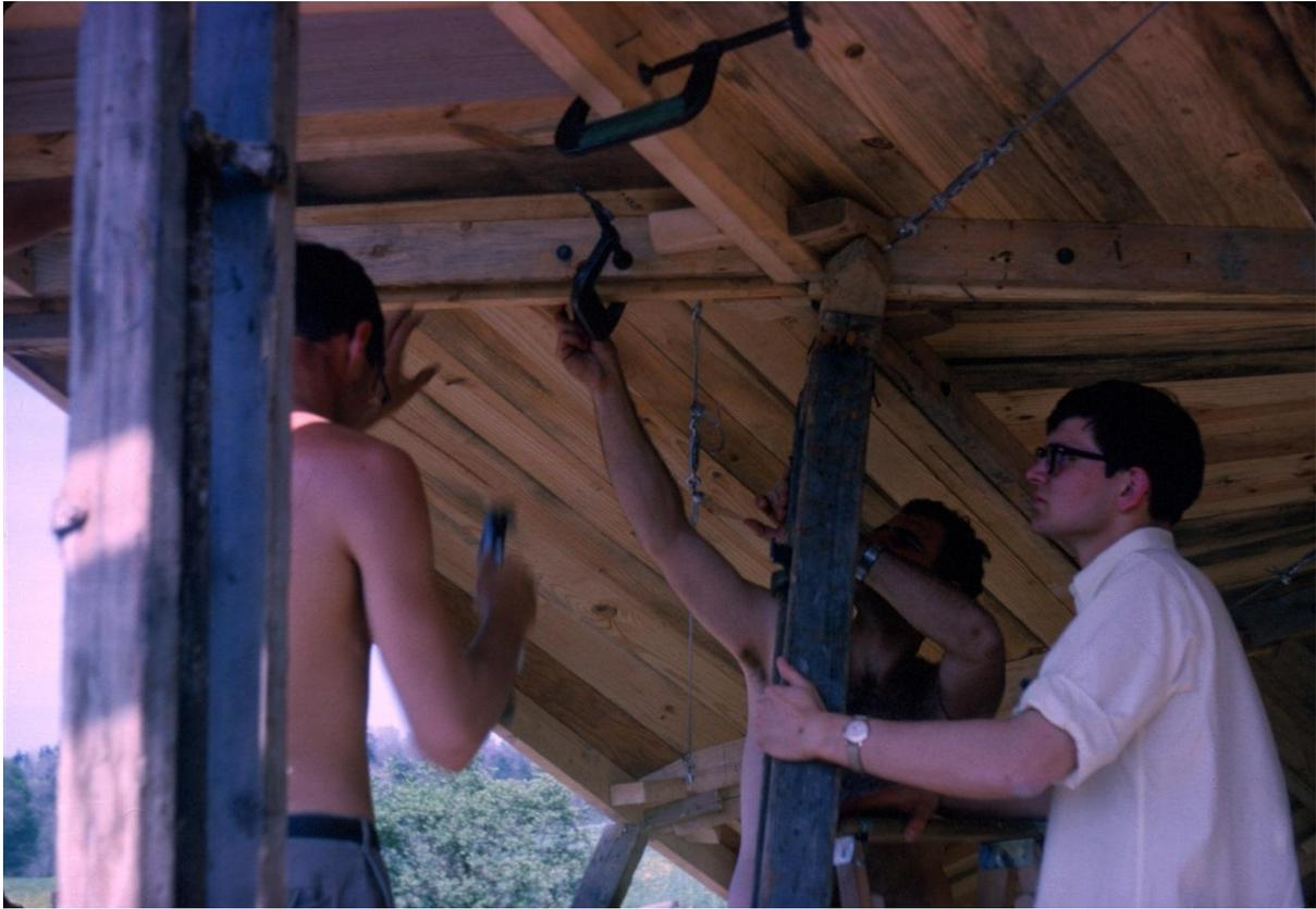
*The sixteen segments of the formwork, built in the basement of Sibley Hall, were bolted together and supported on wooden posts on site.*
