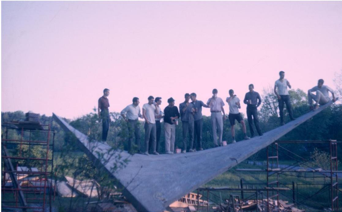
*Eleven of the fourteen students involved in the project and Dr. Greenberg stand on the Hypar. The structure exhibits amazing strength despite being only 2.25 inches thick. The picture was taken shortly after the forms were removed.*
