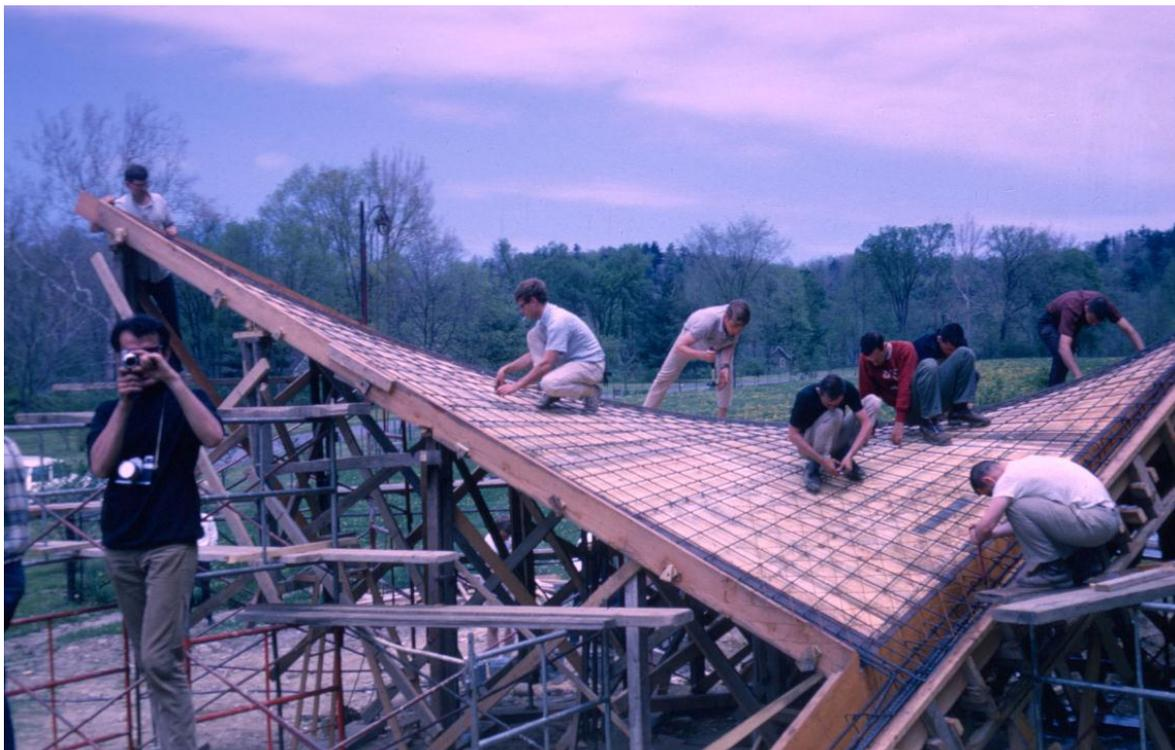
*In this picture, students are preparing the steel reinforcements for the thin concrete shell. Comparing the photo to the previous image one can see that the curved surface can actually be constructed with straight lines. Notice the reinforcing bars at 45-degree angles to the primary curvatures.*
