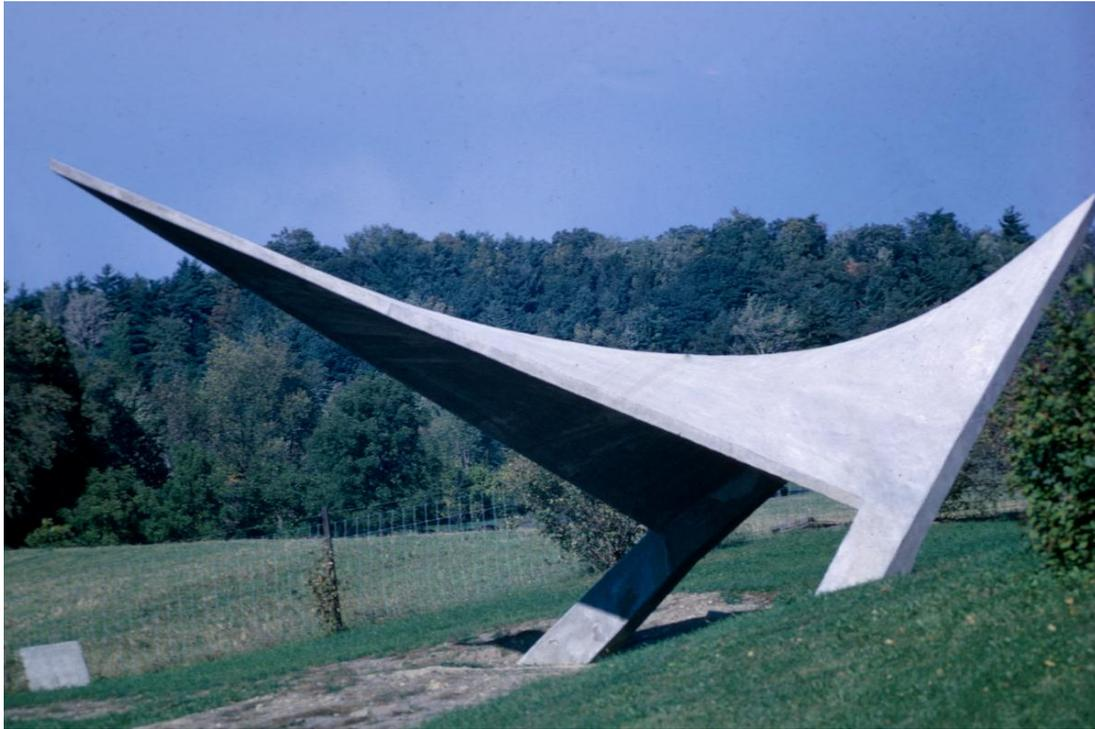
*This photograph of the Cornell Hypar reveals the curvature of the shell. The “anticlastic” surface supports tensile stresses in the hanging direction and compressive stresses in the arch direction.*
